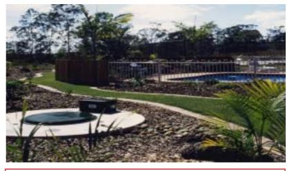
Wastewater and effluent enters the BioCycle by gravity flow through a single inlet drain, then moves through the system's chambers by displacement - i.e. as untreated water flows into one chamber, treated water flows through an outlet into the next chamber, where the water level is slightly lower.
